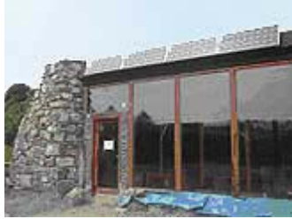
Earthship Fife under construction
