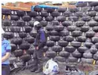
Tyre wall before plastering Earthship Fife
